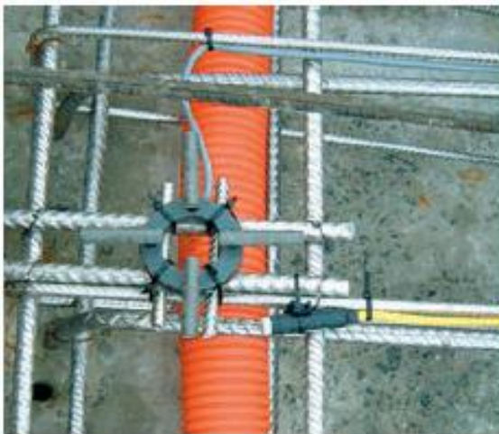
Figure 6: Corrosion cell placed on reinforcement bars before casting concrete.
