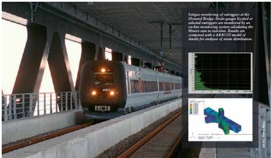
Figure 4: Fatigue monitoring of critical welds by the SHMS on the Øresund Bridge, Denmark - Sweden.
