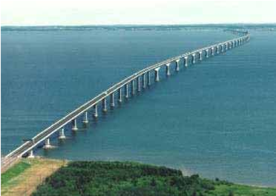
Figure 23: Confederation Bridge – New Brunswick, Canada.
