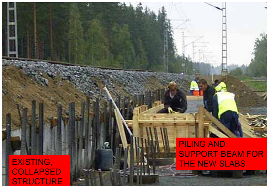
Figure 26: Ermanninsuo construction site, Finland.
