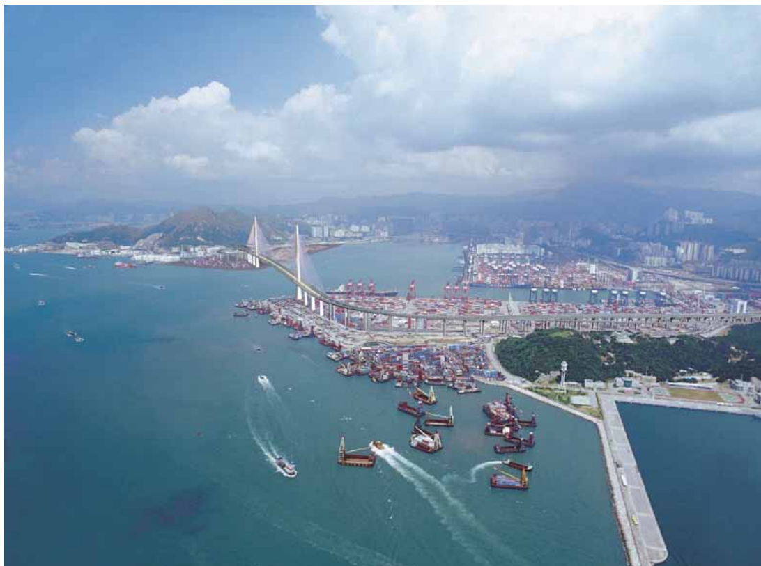
Figure 29: Stonecutters Bridge, Hong Kong, P.R. China. ©Arup.
