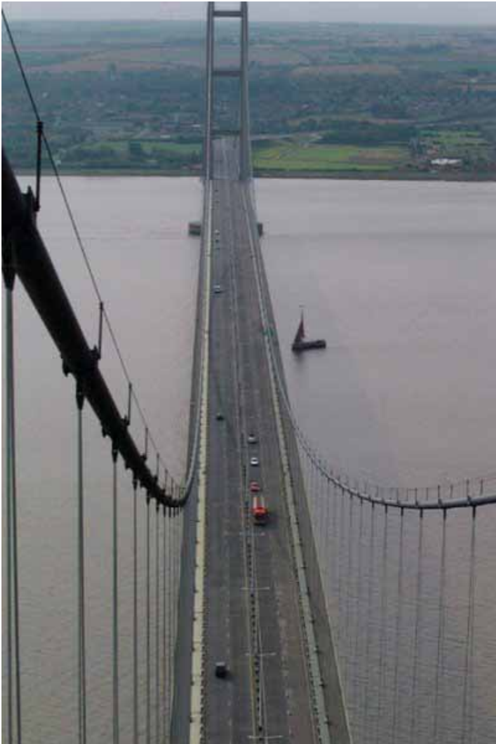
Figure 18: Humber Bridge, United Kingdom
