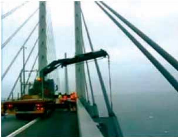
Figure 5: Calibration of FE model by applying a controlled force to a bridge structure.
