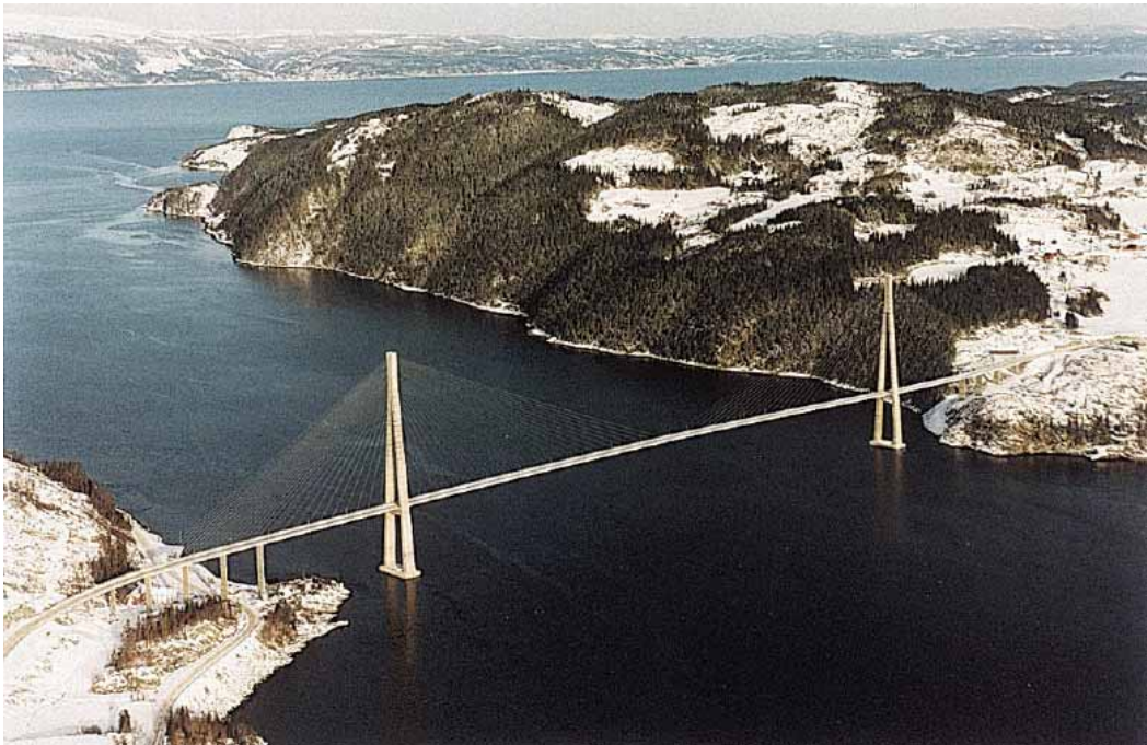
Figure 22: Skarnsundet Bridge, Norway.
