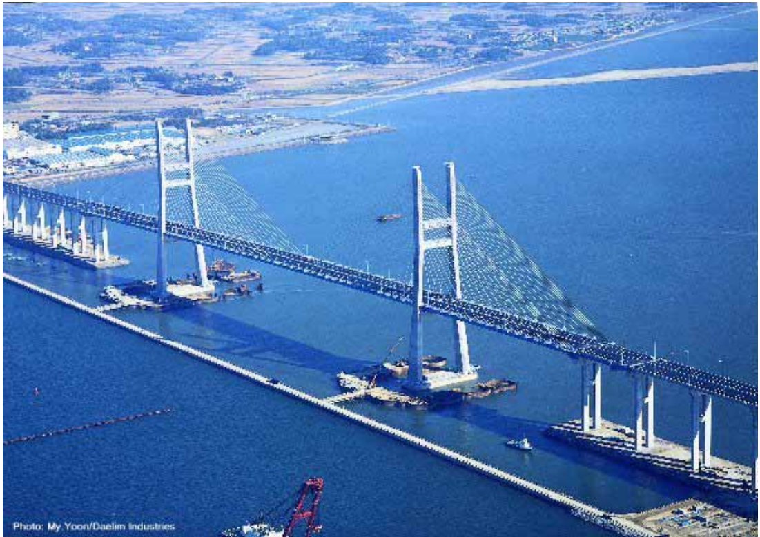
Figure 24: Seo Hae Bridge, Asan Bay, South Korea.
