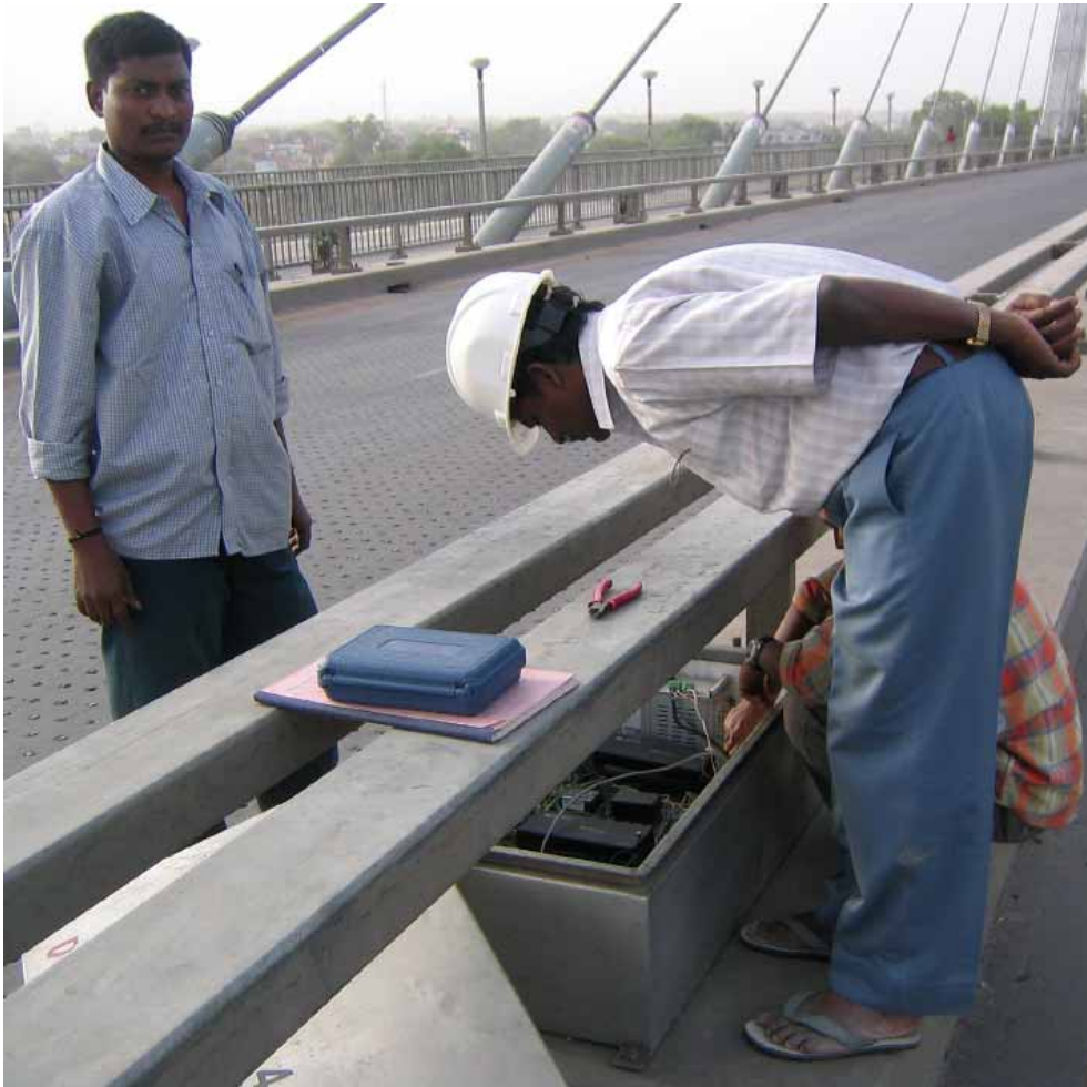
Figure 28: Supervision of SHMS at Naini Bridge, India.
